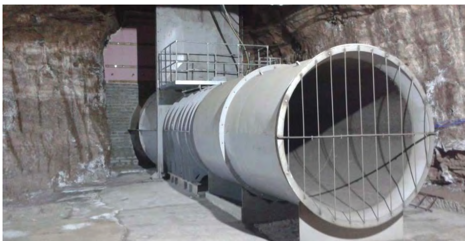
Figure 3. No 1 Zitron Main Fan at Winsford Rock Salt Mine
