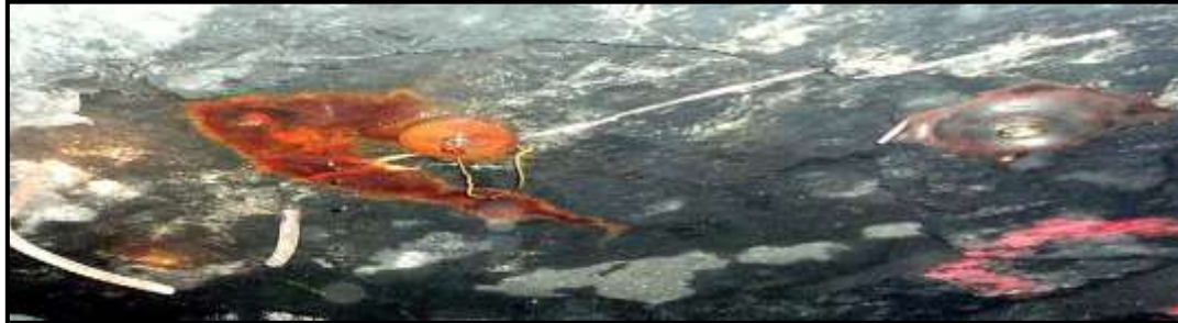
Fig 1. A typical rock bolt deterioration due to corrosion.
