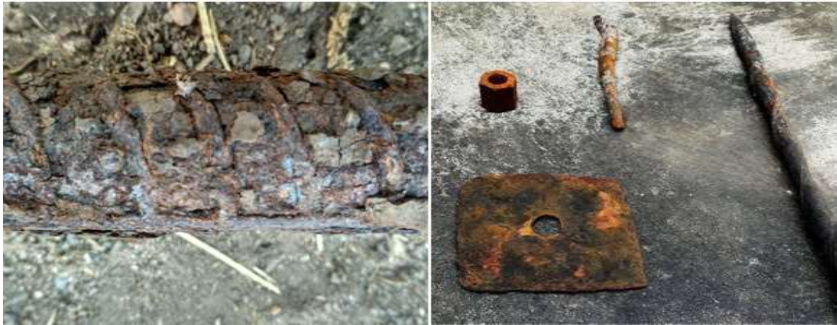
Figure 1 - Fully corroded rock bolt sample from mine A
