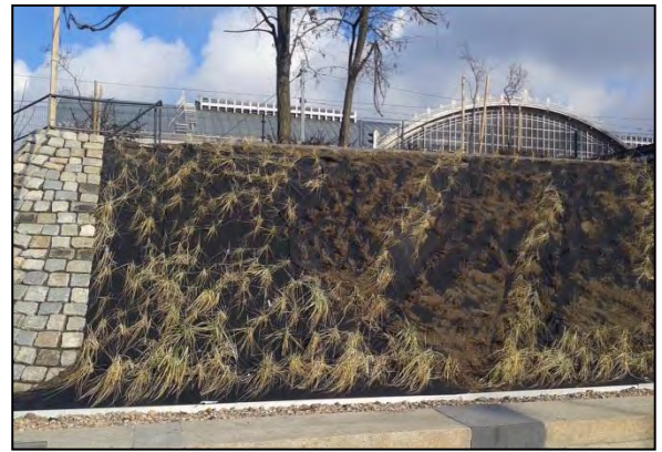
Figure 2. Slope of the embankment of the main railway station in Wrocław city. The combination of grass and mat. Photo M. Spitalniak
