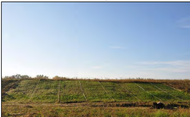
Figure 6. Slope of 8 test plots, the plots are separated: plots with geocomposites and control plots. Examines the effectiveness of geocomposite depending on the depth of the foundation. Photo M. Spitalniak
