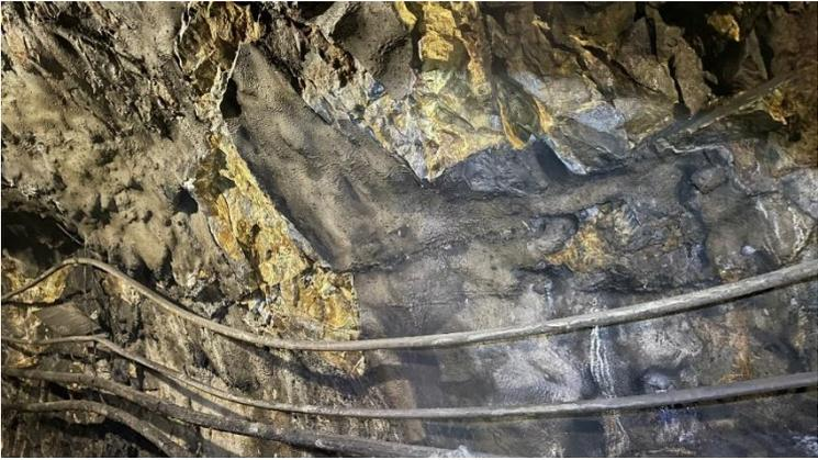
A photograph of a mine shaft wall showing a distinct horizontal layer of rock that has delaminated from the main rock mass. The delamination is most prominent in the center and right side of the image. The rock is dark and appears to be a different type of material, possibly a contact zone. There are some cables or pipes visible in the foreground. |
