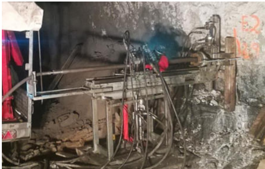
Figure 10: Small scale underground core drilling rig
