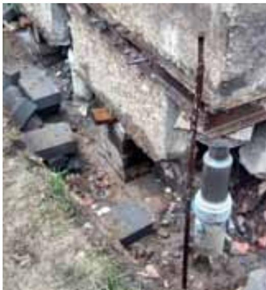
Figure 1. Lifting the building with hydraulic jacks
