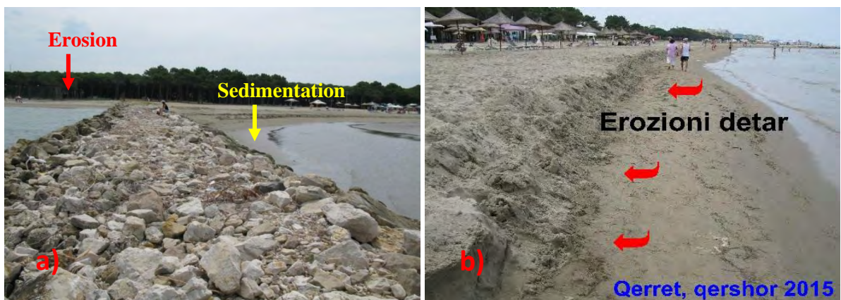
Figure 3. a) Groin which prevent the movement of sediment and on one side have sedimentation and on the other side have erosion, b) Sea erosion of the coastal line
