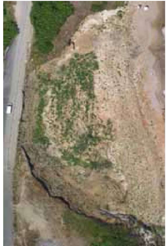
Fig. 1. Orthophoto mosaic of the landslide above the Alepu beach.
