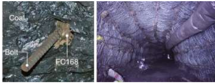
Fig. 3 Detailed show for fully bonded bolt and photo for section supported by fully bonded bolts
