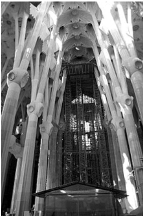
Biomorphic branching columns in Gaudí's monumental but still incomplete Sagrada Família church are modelled on trees
