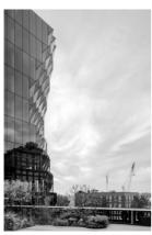
Studio Gang, the Chicago-based architecture firm, designed the 139,000-square-foot building using a strategy it describes as "solar carving." The architects mapped the sun's annual course to determine which parts of the nearly finished 12-story tower to slice away and sheathed portions of those sections in tilted angular panes of glass.
